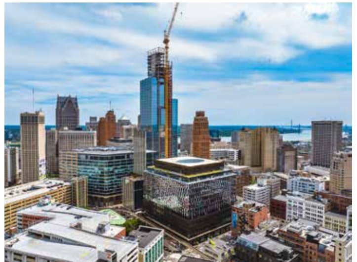
The tower under construction with the office building in the foreground
