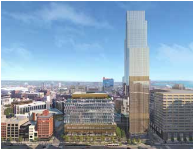
(l-r) The office building and the tower at Hudson's Detroit
