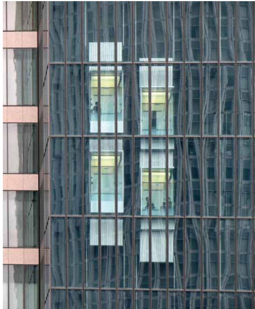
Representative double elevator (at Midland Square, Nagoya) 双层电梯的代表 (米德兰广场, 名古屋)
